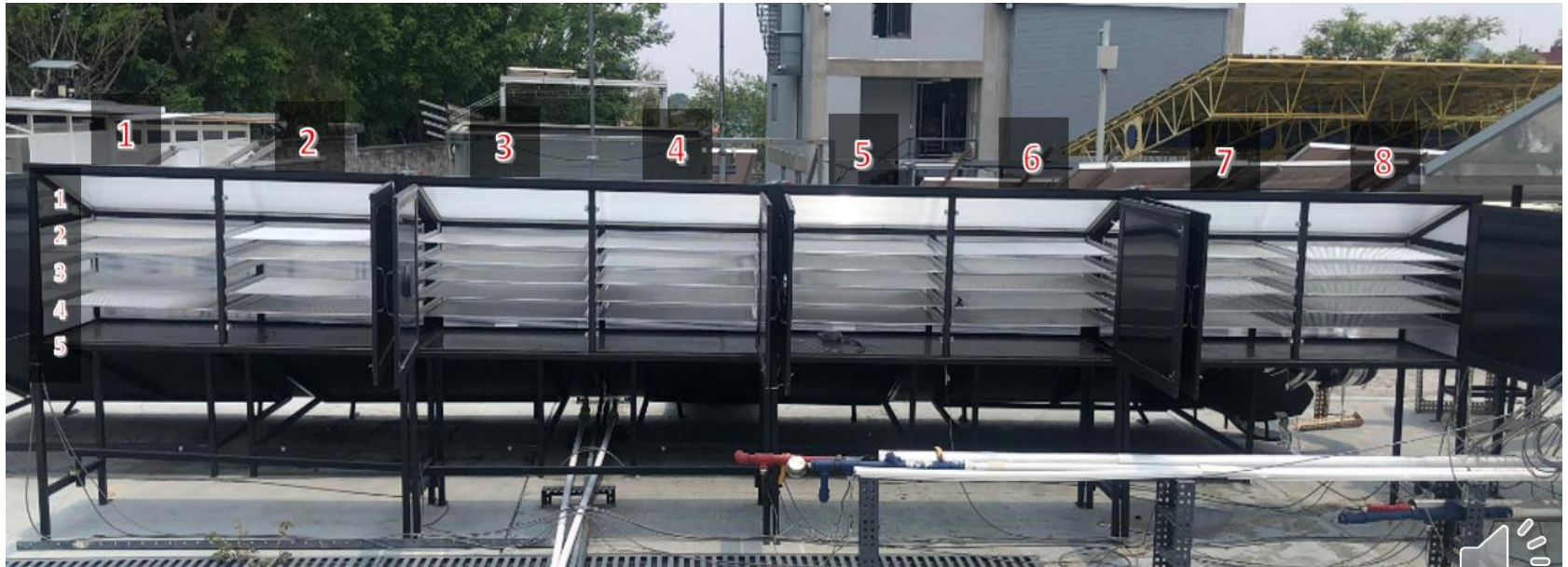
Figure 8 Distribution of trays in the drying tunnel
